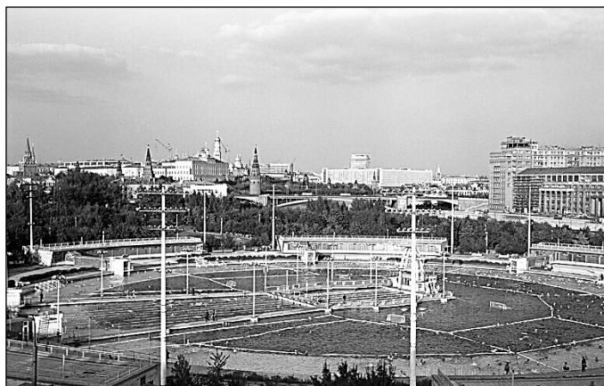
Figure 172: The giant open-air “Moskva” swimming pool that occupied the site of the demolished Cathedral of Christ the Savior from 1958 to 1994. Built in the foundation pit left after the 1931 dynamiting, the pool stood on the site until the land was returned to the Russian Orthodox Church for reconstruction in 1994. (Photo: Russia Beyond , 2011. Reproduced for educational/scholarly purposes only under fair use.)
