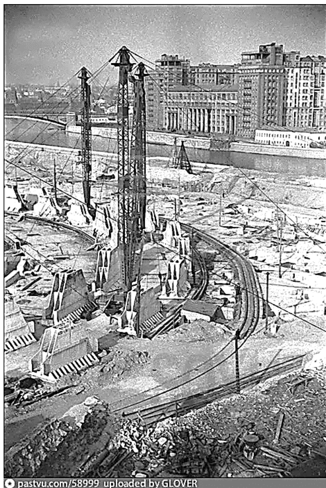
Figure 170: Moscow, 1938. The ill-fated concrete foundation for The Palace of the Soviets flooded continuously and was never robust enough to carry the weight of this modern-day Tower of Babel. Thank God. (Photo: pastvu.com/58999 . Fair Use.)
