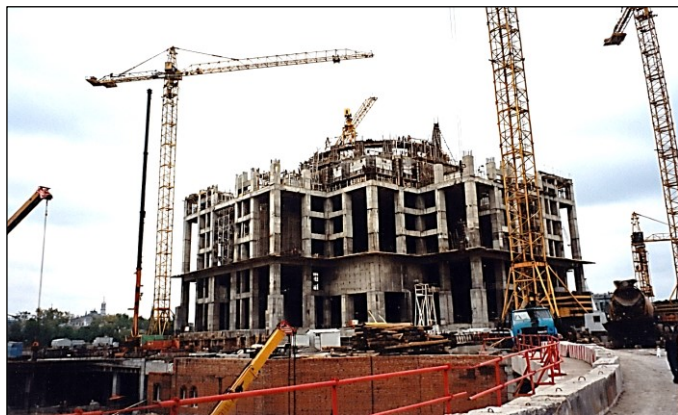
Figure 174: The Cathedral of Christ the Savior under construction in Moscow, September 1995. This was our view as we walked up the ramp on the right. The massive concrete and steel shell of the new cathedral rises on the site where the original church had been dynamited by Stalin in 1931. Cranes and scaffolding surround the structure during the early phase of rebuilding, just days before the historic cross procession on September 7, 1995 in which the OCA delegation were honored guests. (Photo: Stephen Gidus, also a delegate (1995). Fair Use. McKibben archive.)
