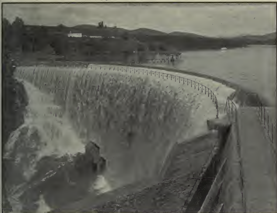
The famous Sweetwater Dam, built of solid masonry 120 feet high.
